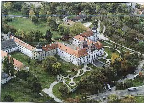
Aerial view on the Royal Palace
